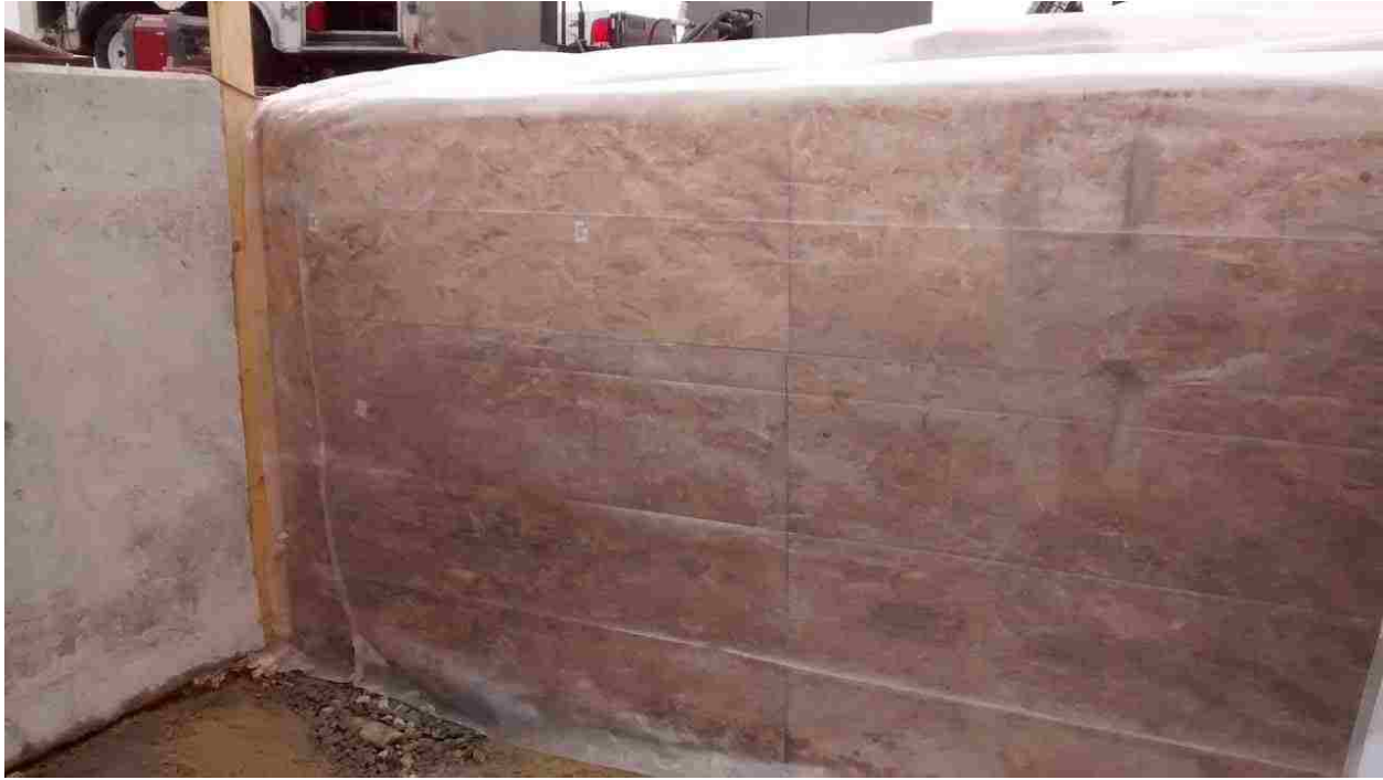
Figure 3-5. Box side wall covered with plywood and first layer of plastic.
